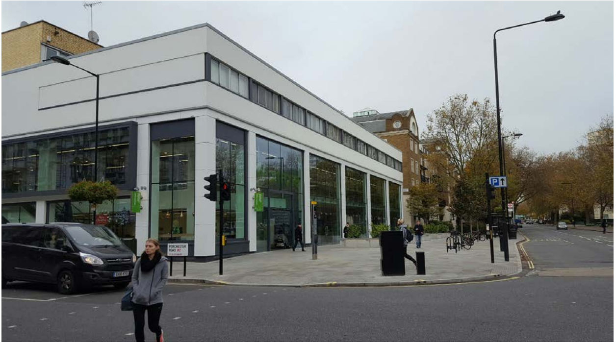
View from corner of Bishop's Bridge Road and Porchester Road.
